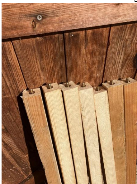
Top of the legs prepared with fixings
