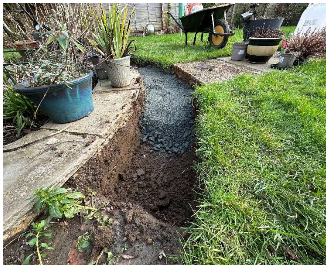
Track bed being constructed
