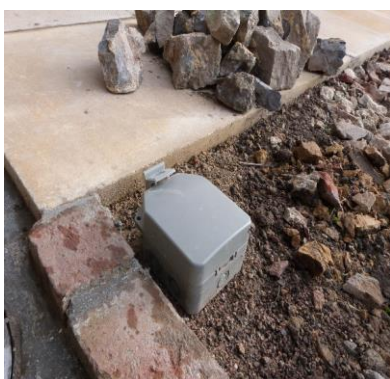
One socket installed
