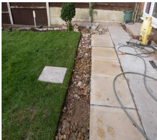
Track bed dug out with hard core in place awaiting concrete
