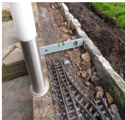
Levelling the track bed and ensuring clearance for small wall
