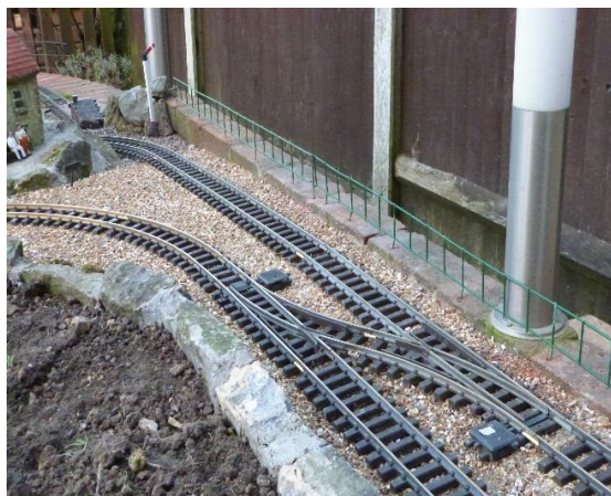
Safety fencing running along the top edge of the wall
