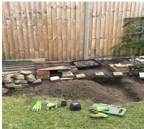
Repair work and a new way forward
