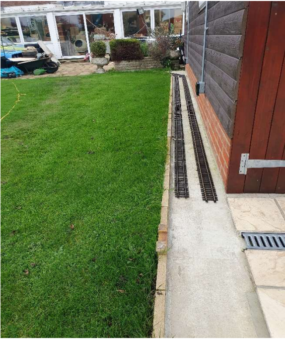
Track on the Righthand side with part of the track laid
